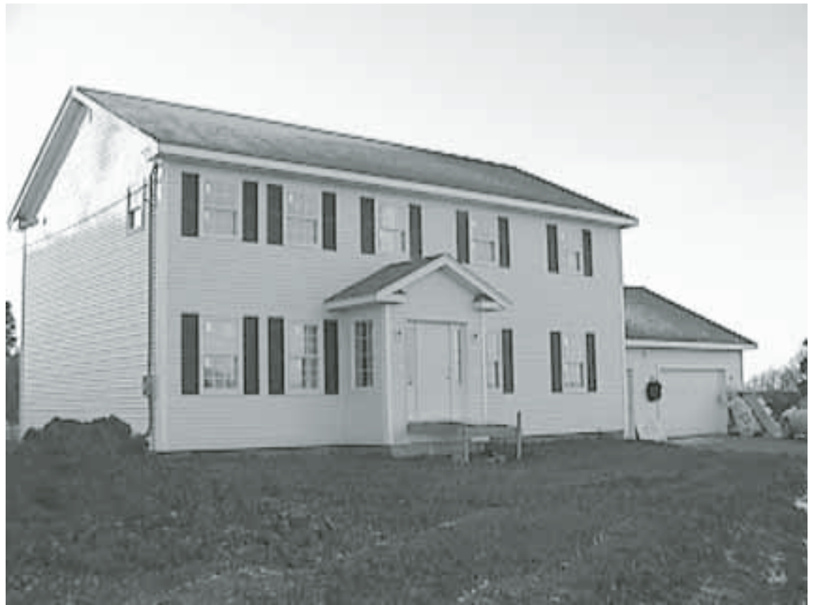
This new rectory for the Parishes of Waterford and St. Mark is built to diocesan standards with four bedrooms, two and one-half baths, kitchen, dining room, living room, family room, laundry room, rector's study, plenty of storage space and a garage.
