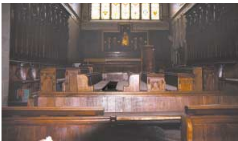
The remodeled and now comfortable pews had to be stored somewhere while the new floor was installed. The choir stalls, chancel, sanctuary and lady chapel were pressed into service
