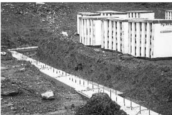
A new church for Richmond Corner under construction for the Parish of Richmond began to take shape in late August when the first concrete was poured. The church and its hall are being constructed of ICF (Insulated Concrete Forms), making it very heat and energy efficient. Ground water heating will also cut down on energy costs. The buildings will replace St. John's Church, which is 136 years old this year.
